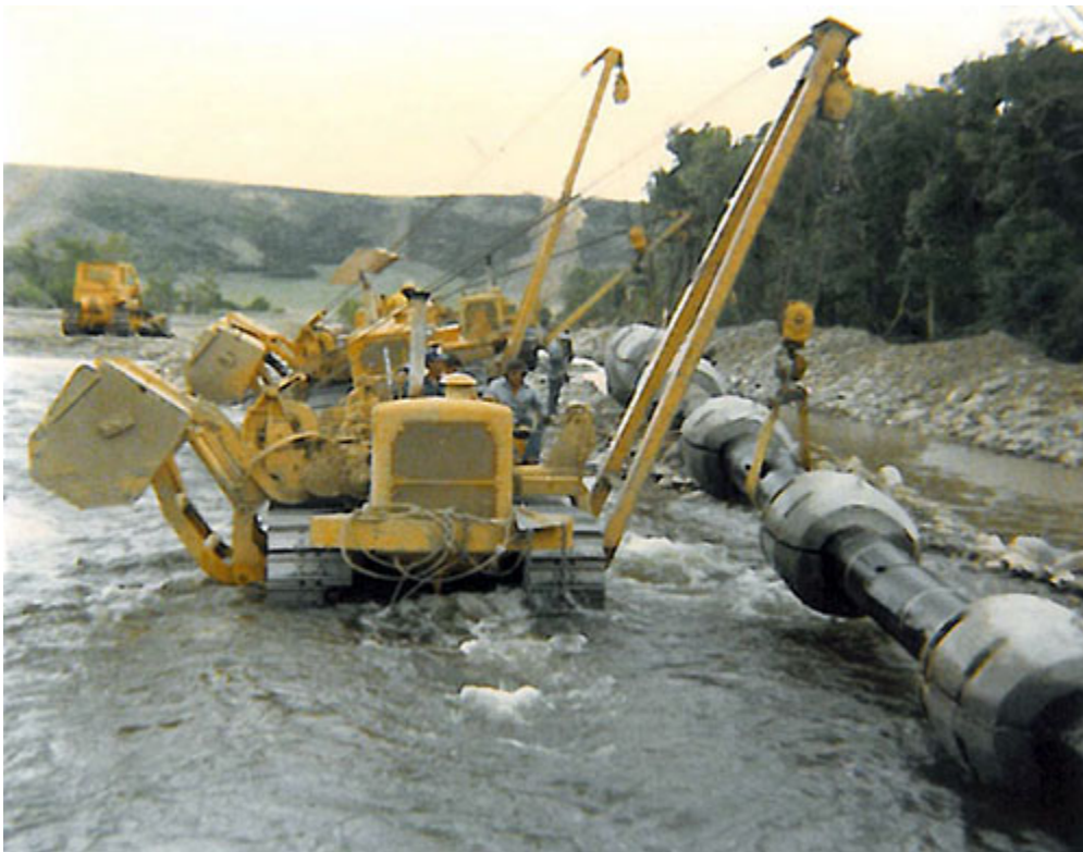
(1970s construction on the Rawlins-Hesston line.)
